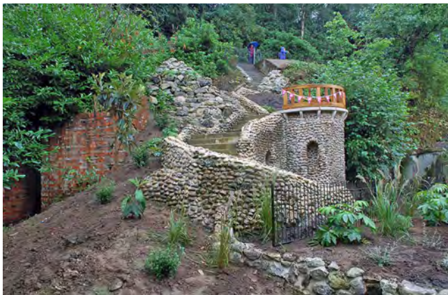
The Embattled Tower folly is flanked by three sealed entrances to Howard's tunnels and the WWII bunker
